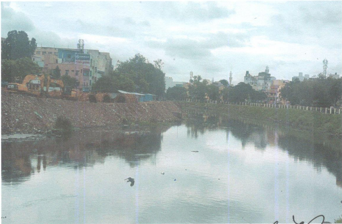
Pier – P106 to P109
