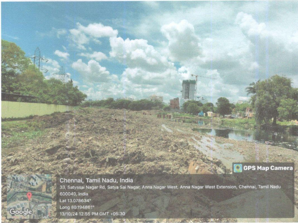
Pier – P437 to P439
