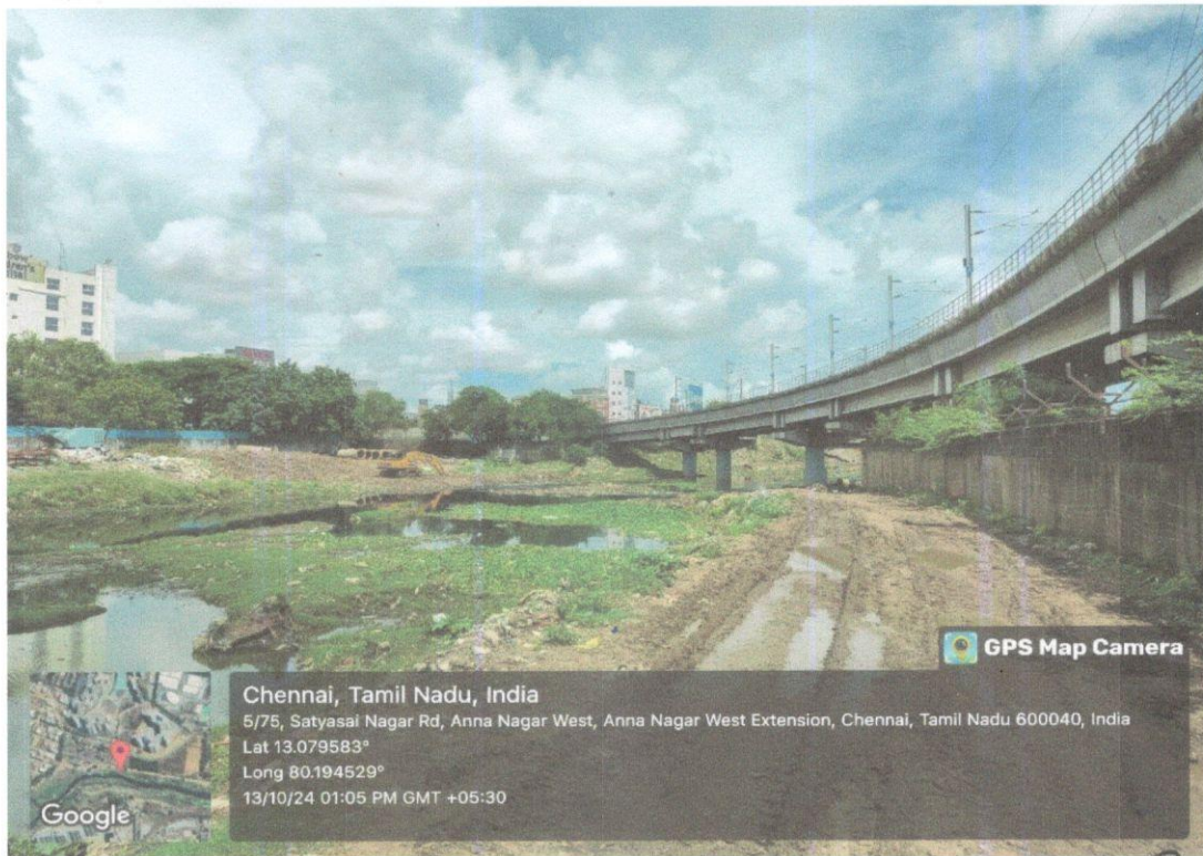
Pier – P428 (River Crossing)
