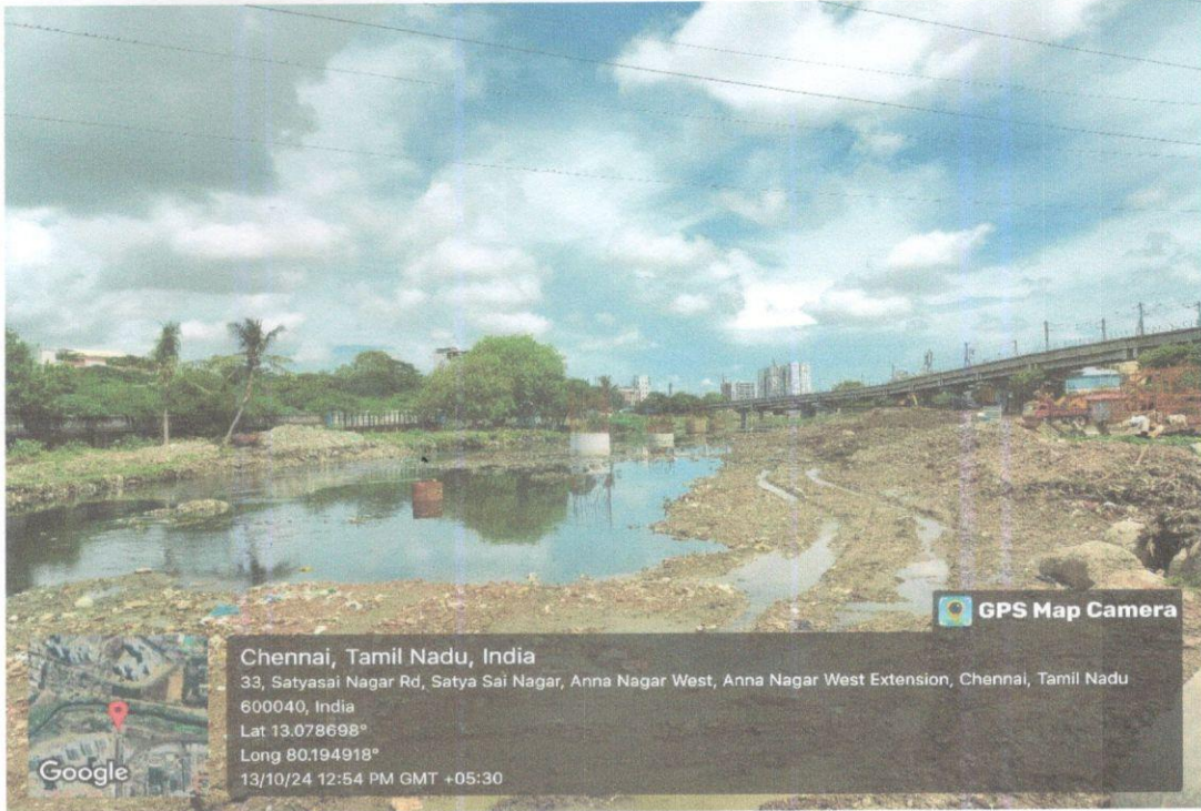
Pier – P431 to P435
