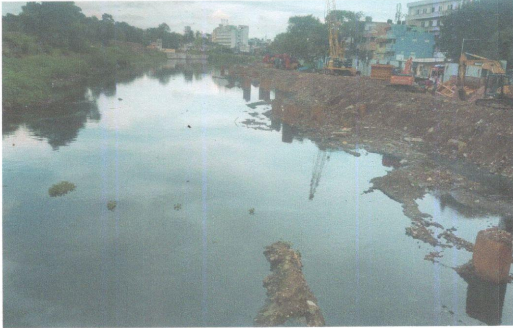
Pier - P75 to P85
