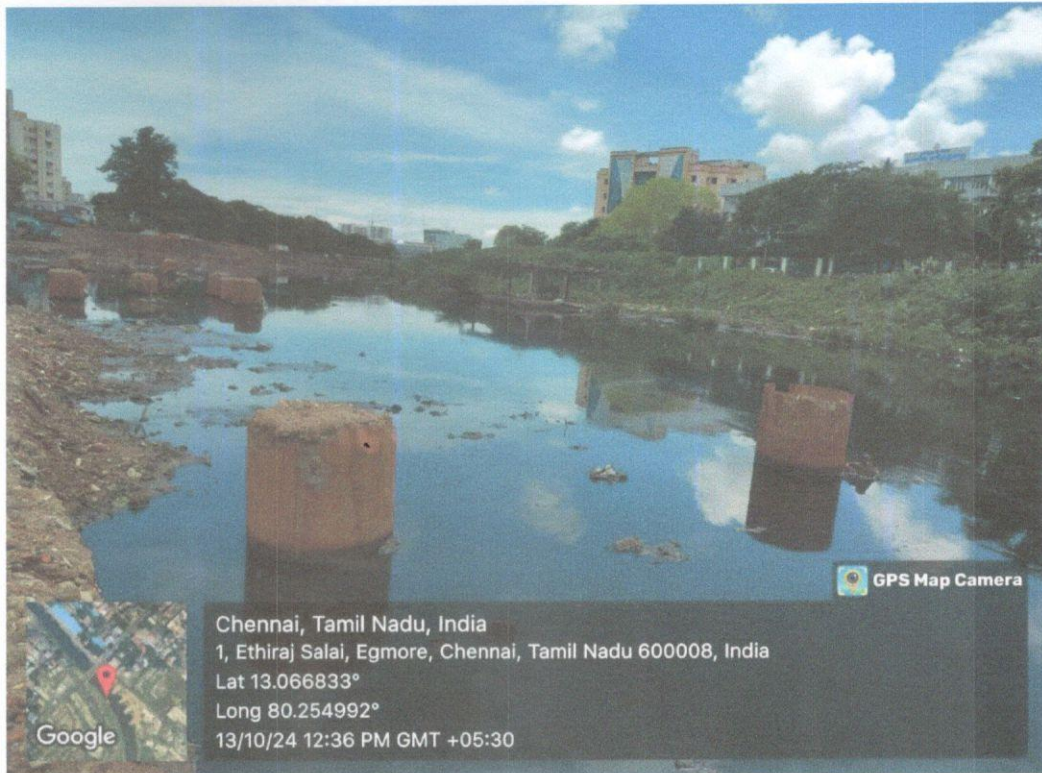
Pier – P175 to P177
