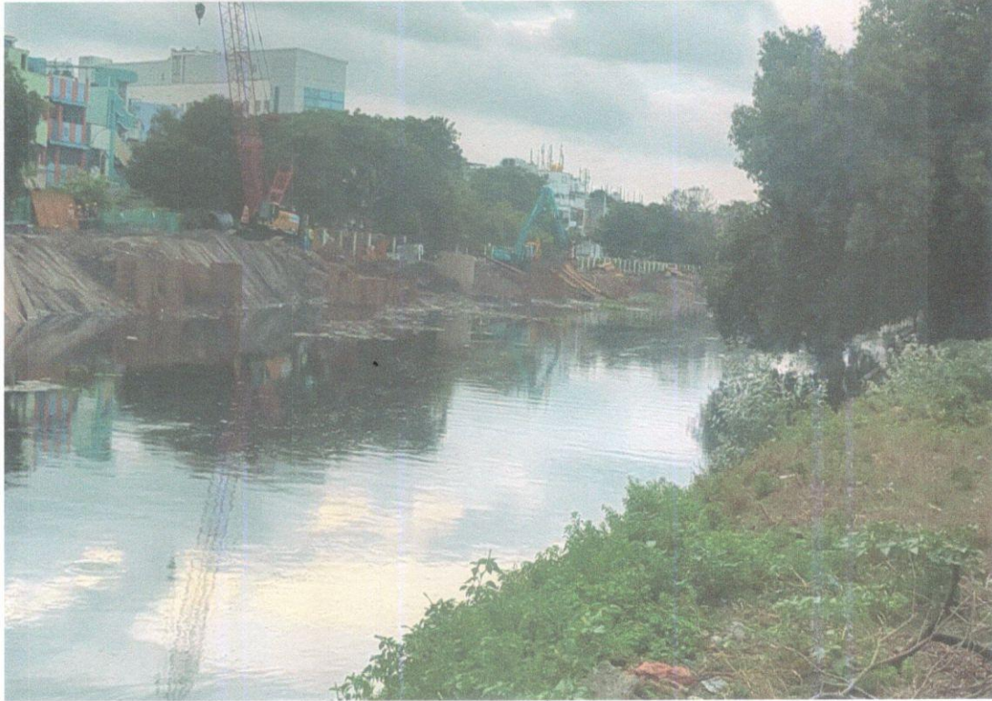
Pier – P100 to P103
